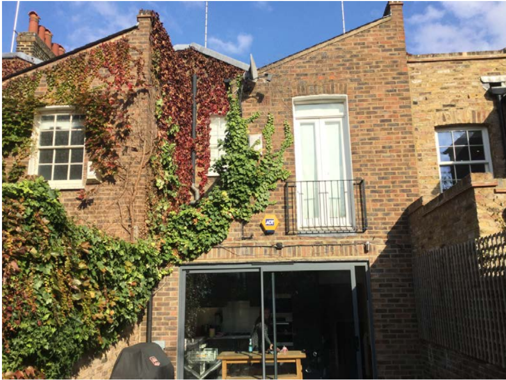
Rear elevation of 62 Bourne Street
